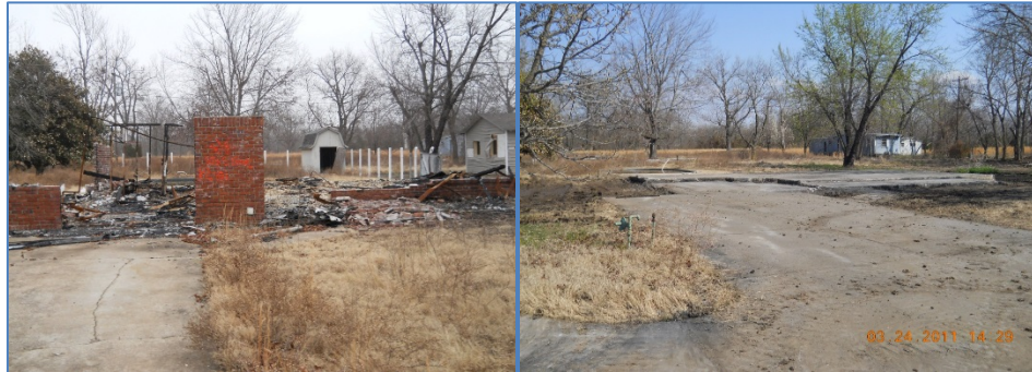
103 S. Ethyl – Before Demolition 103 S. Ethyl – After-Demolition
